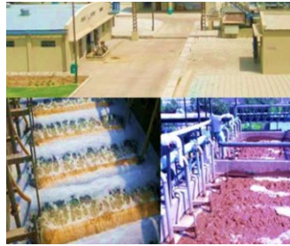
Common Effluent Treatment Plant
