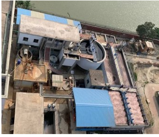
Membrane Bio Reactor (MBR) Based Effluent Treatment Plant (ETP)
