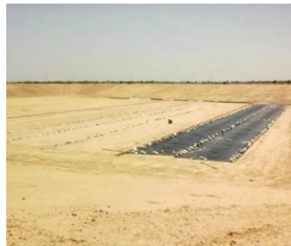
Secured Landfill Site for Disposal of Hazardous Waste
