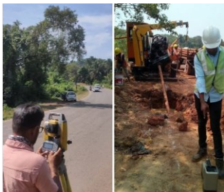
Trenchless Sewerage Network for Urban Development Authority
